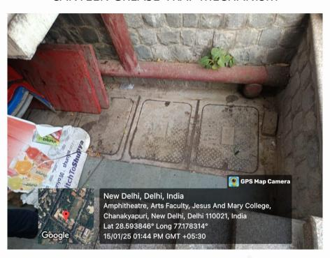
3 compartment grease trap system to filter heavy particulate matter, grease and waste water from canteen drainage.
